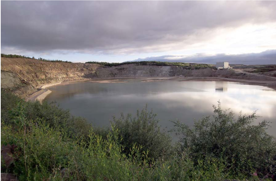
Figure 1.1-5: Rabbit Lake In-Pit Tailings Management Facility (RLITMF).
