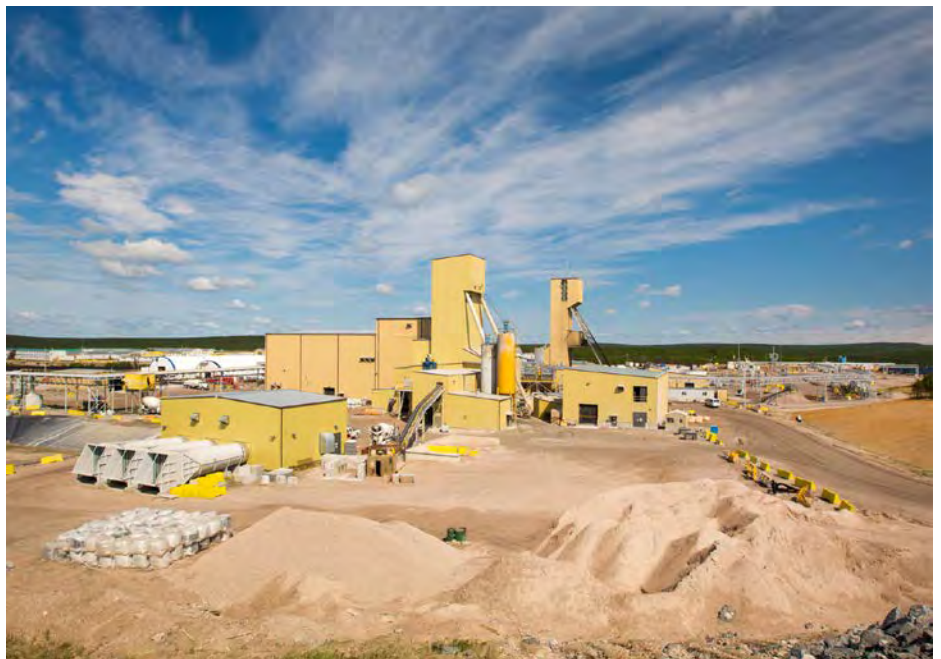
Figure 6 Cigar Lake Uranium Mine, Norther Saskatchewan, Canada Source: Cameco Corporation
