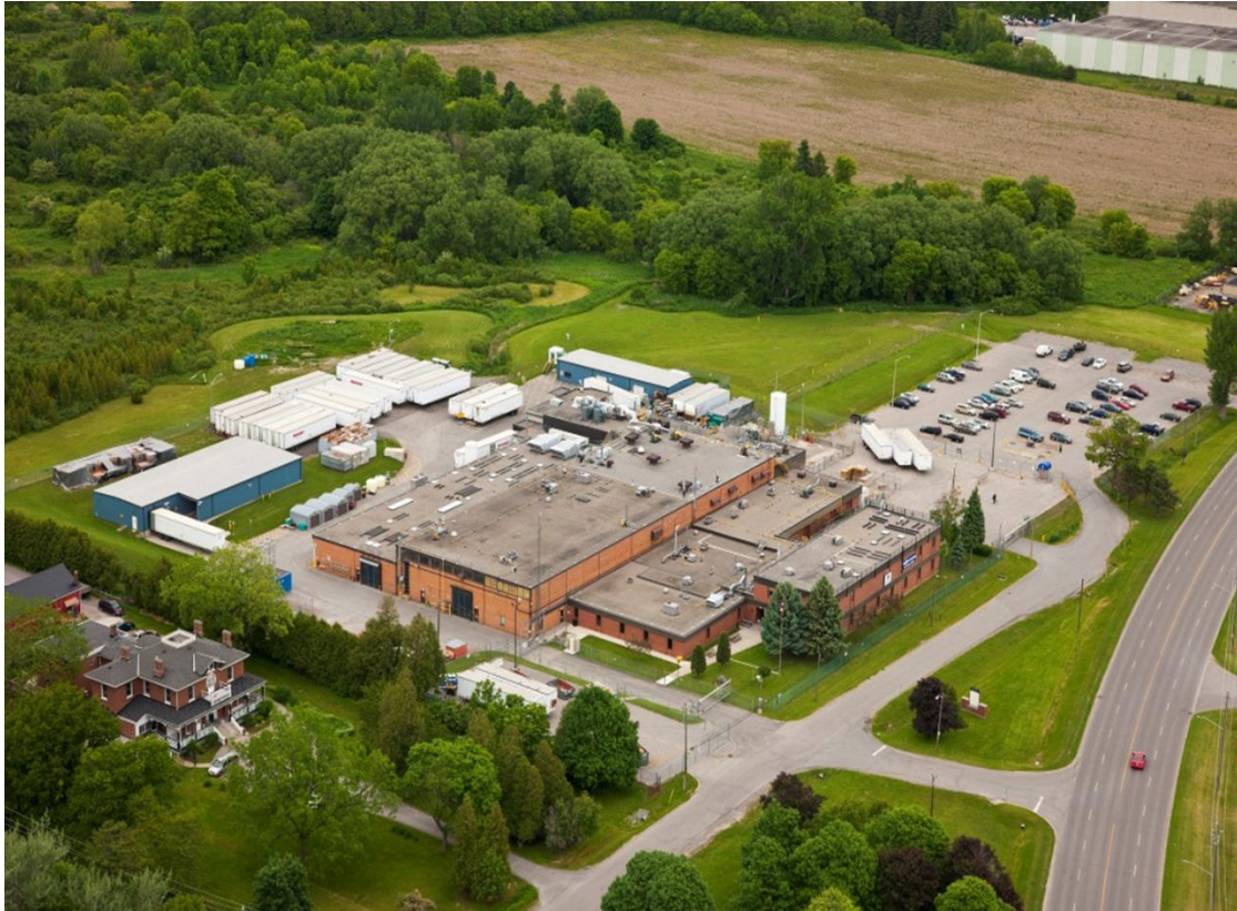
Figure 2 – Aerial View of Cameco Fuel Manufacturing
